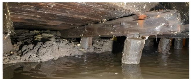
Fig. 1: Timber Piles of the Foundation
