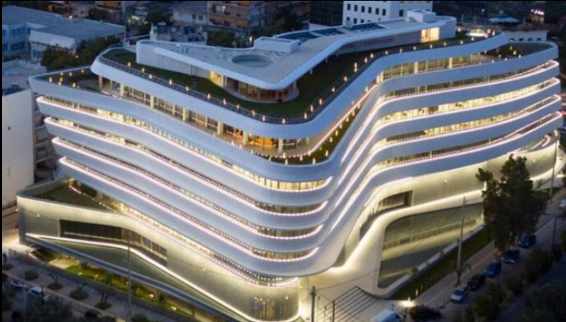
Aggemar Office Building SA EcoStruxure Power & Building Solutions
