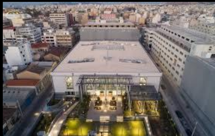
Piraeus Port Plaza Complex EcoStruxure Power & Building Solutions
