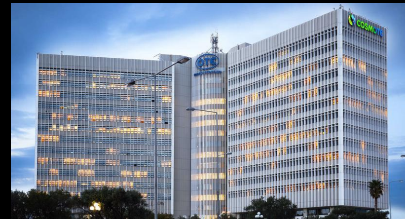
OTE Building EcoStruxure Building Solution Renovation
