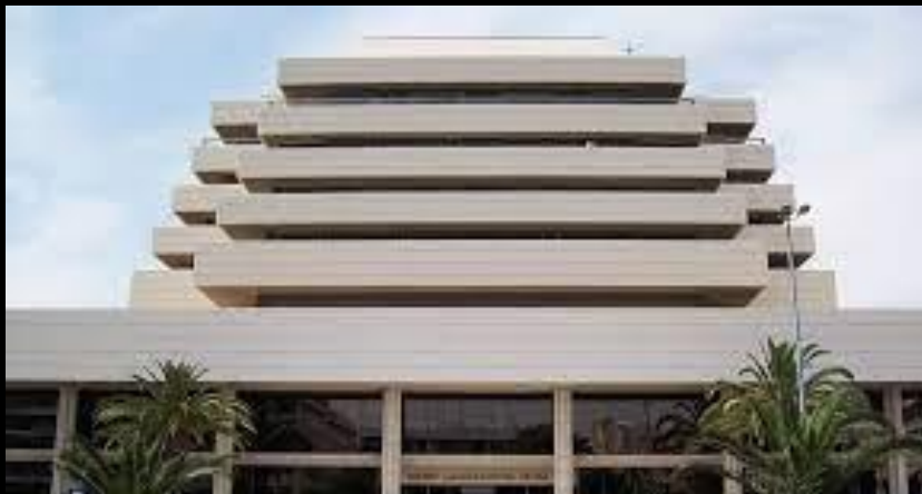
Onasio Hospital EcoStruxure Power & Building Solutions
