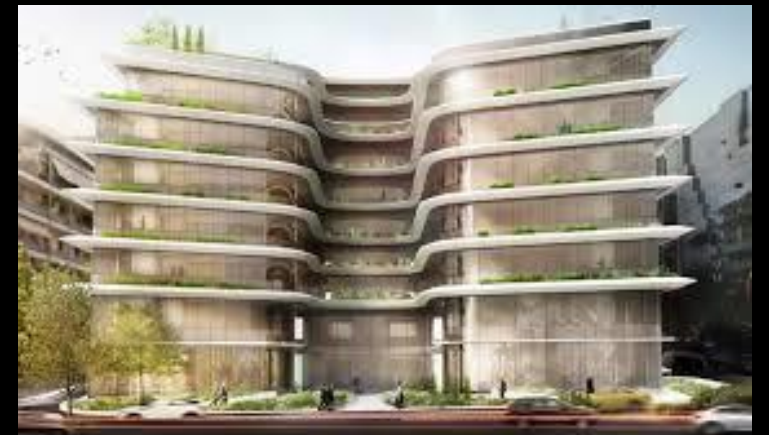
Orbit Office Building EcoStruxure Power & Building Solutions
