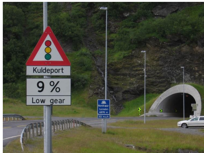
The mainland entrance to the North Cape Tunnel. Konrad Zielinski / Wikimedia Commons
