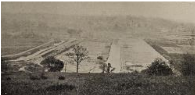
Image 20: Cutoff trench (center) of the Huffman Dam near Fairborn, OH, in the Miami Conservancy District during its construction, late 1910s. Source: Baker et al. (1923).
