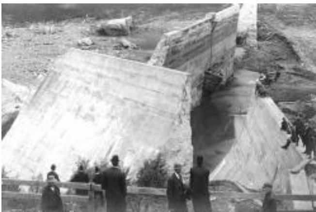
Image 18: Onlookers take in the remnants of the Austin Dam after its failure, fall 1911. Source: Kline et al. (2021).
