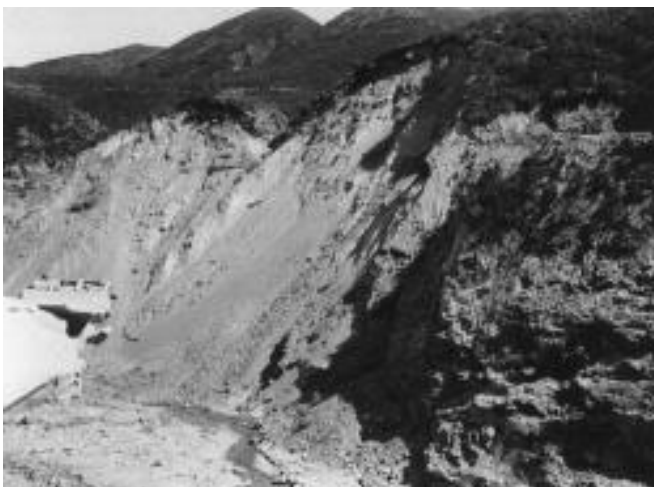
Image 14: Close-up of the east abutment landslide at the St. Francis Dam site following the breach. Source: Rogers (1995).
