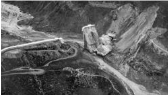
Image 1: Aerial view of the St. Francis Dam's remnants after its March 1928 breach. Source: Harrison (2018).
