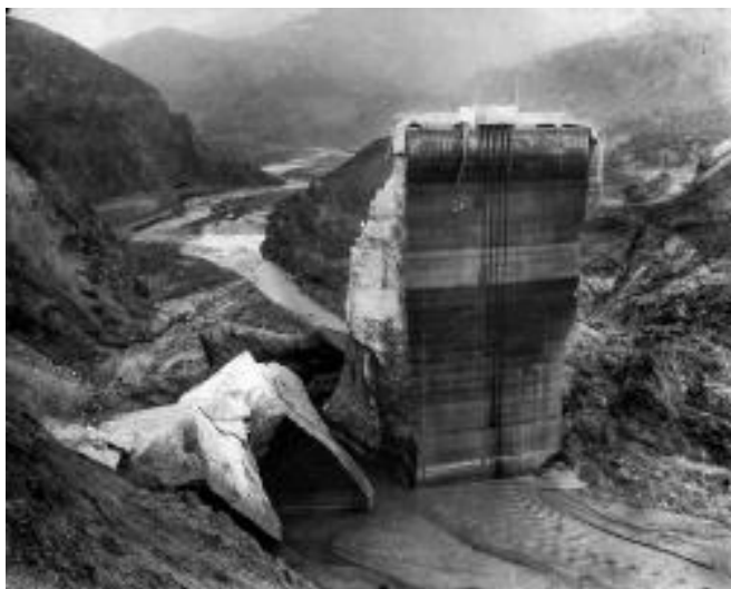
Image 23: The St. Francis Dam remnants shortly after the structure's breach, March 1928. Source: Harrison (2018).
