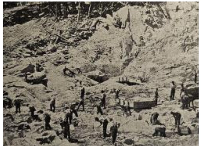
Image 15: Early stages of foundation excavation at the Arrowrock Dam, mid-1910s. Source: Baker et al. (1923).
