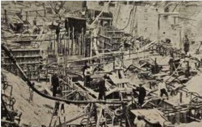
Image 11: Hoses for well point dewatering snake through the excavation for the Ritz-Carlton Hotel in Atlantic City, NJ, c. 1920. Source : Baker et al. (1923).
