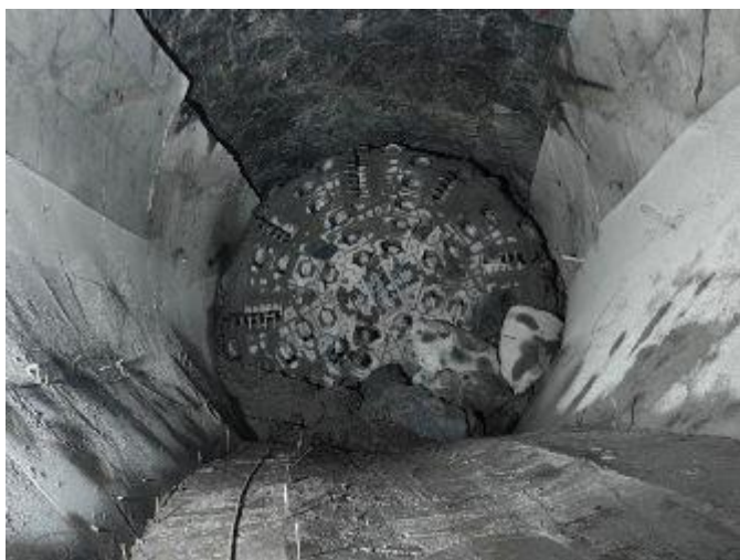
The Breakthrough of "Tianyue" TBM
