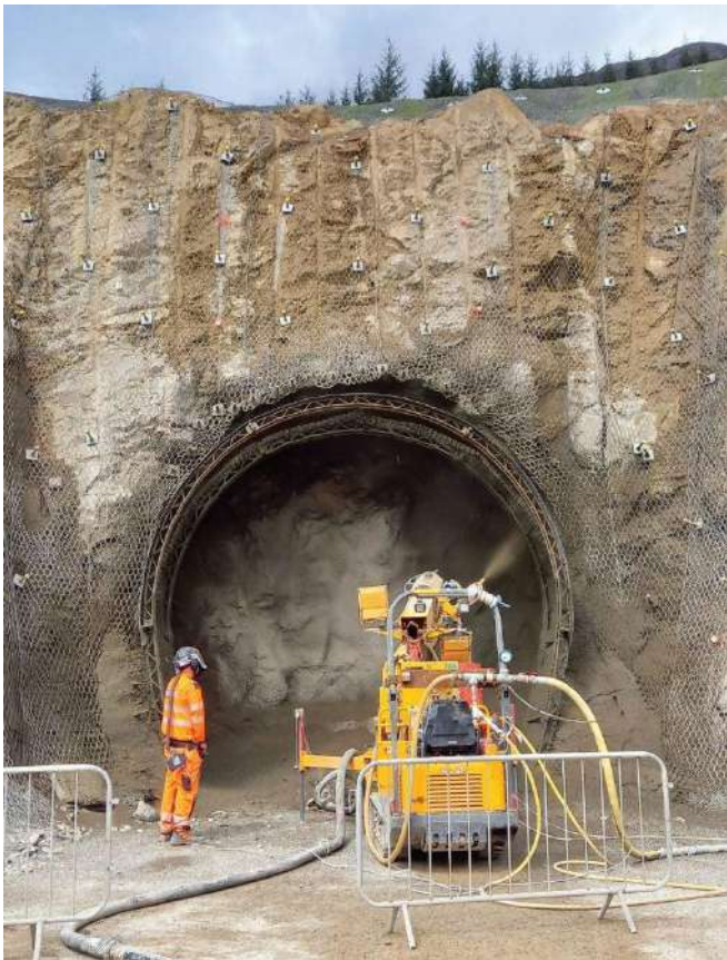
Adit portal construction PHOTO CREDIT: JOE COXSON
