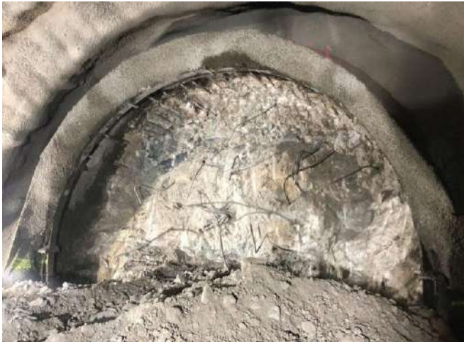
Steel ribs and Class-SQ top heading excavation, respectively PHOTO CREDIT: JOE COXSON
