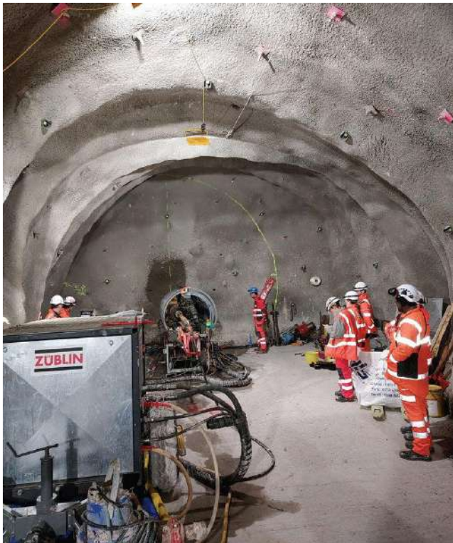
Zublin setting up for drilling at the fault zone PHOTO CREDIT: TOM ROBINSON
