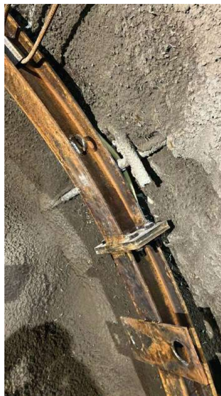
Steel ribs and Class-SQ top heading excavation, respectively PHOTO CREDIT: JOE COXSON
