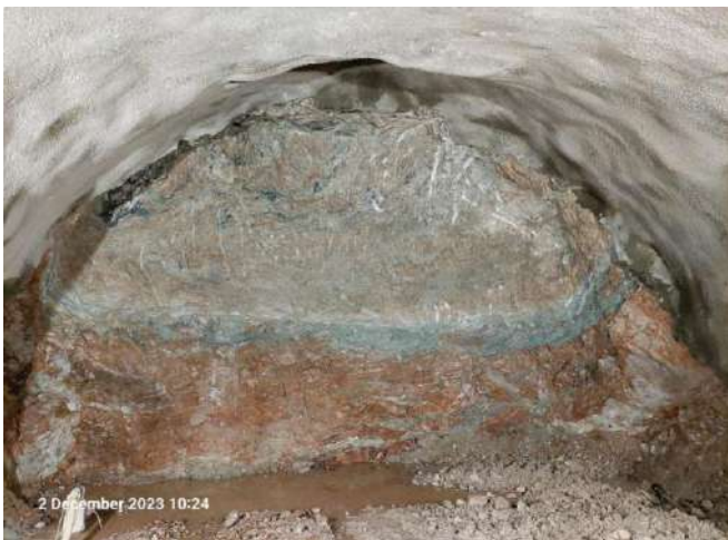
Photo of exposed geology and corresponding face mapping sketch at Advance 284 of the Adit PHOTO CREDIT: ANTONIA DECMAN
