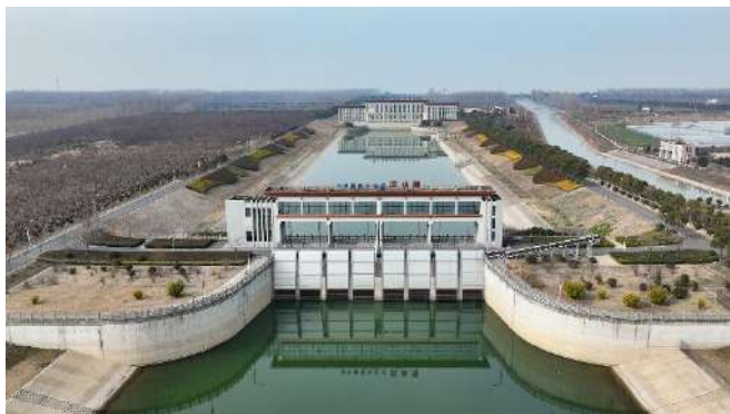
The Hongze Station on the eastern route of the South-North Water Transfer Project in Huai'an City, China. (Image credit: CFOTO via Getty Images)
